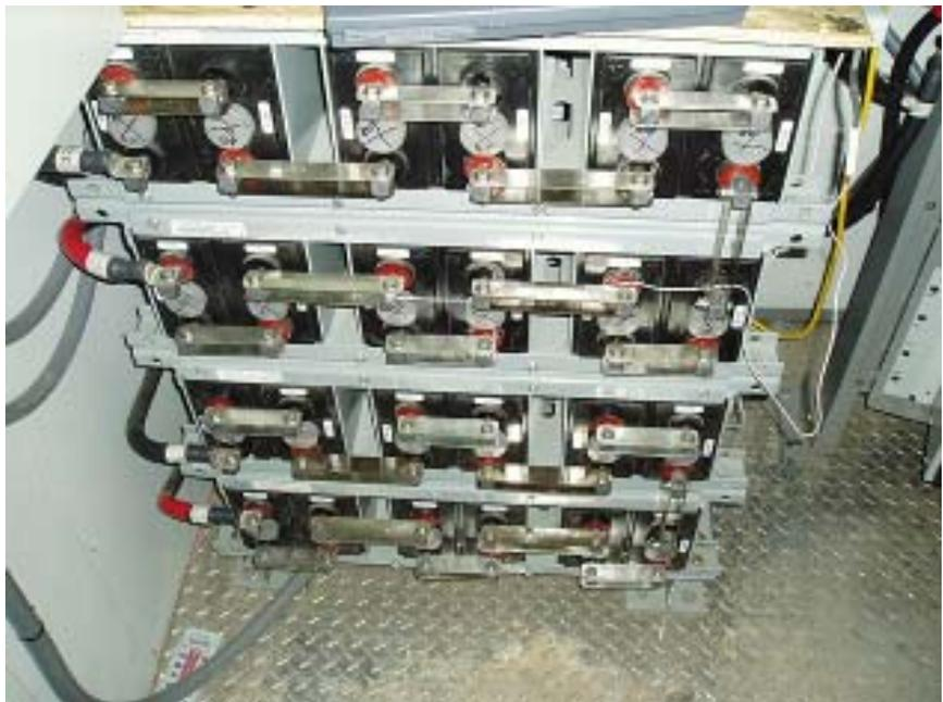
*Industrial battery stacks offer the ability to reconfigure voltages based on 2 volt cells. They can also allow for a lot of energy storage in a compact space.*
