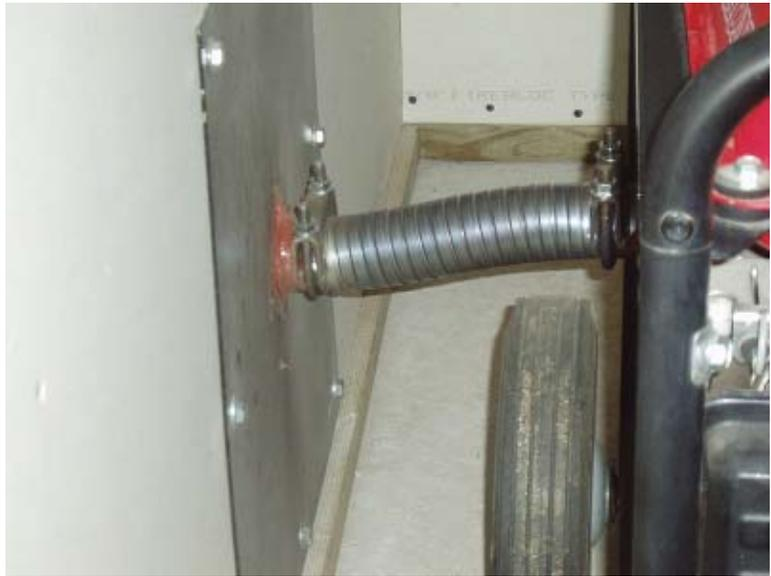
*Combustion exhaust gases are poisonous and very hot (>500F). Penetrations in enclosures must be properly designed for safety and reliability. Note the large flange and flexible, high-temperature connector pipe.*
