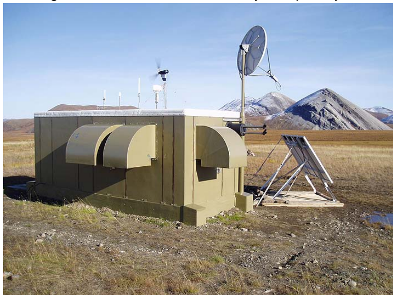
The module after installation of wind and solar components.
