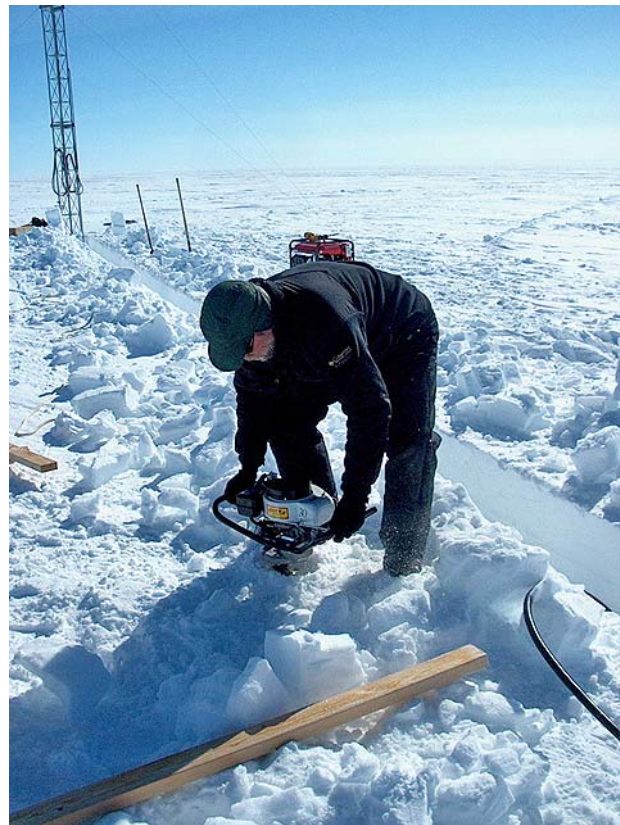
Tracy Dahl drilling a 4 x 4 post for solar panels.
